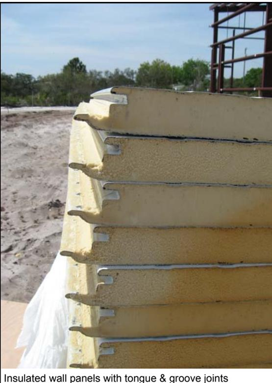
Insulated wall panels with tongue & groove joints
